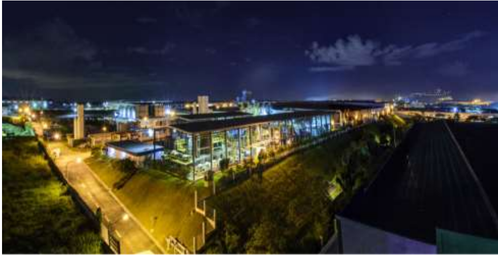
Figure 2.4 Industrial Land Offering inside FPIP
