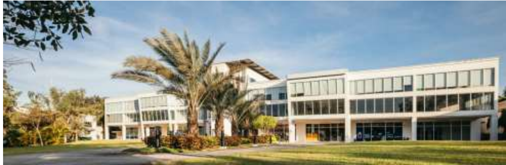
Figure 2.7 Oasis Commercial Centre Offering inside FPIP
