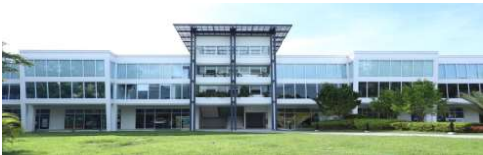
Figure 2.8 Socio Civic Building Offering inside FPIP
