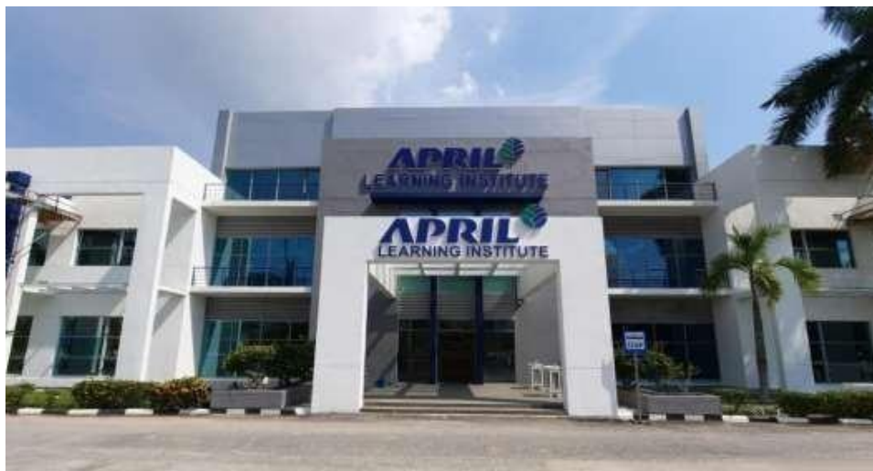
Figure 2.7 ALI Building Source: Internet
