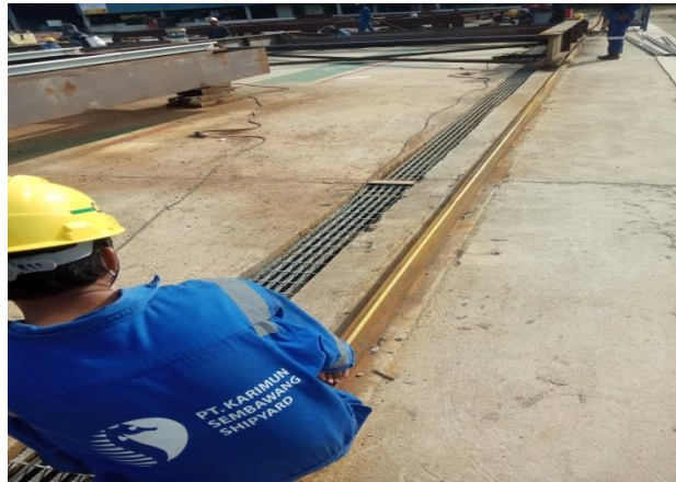
Gambar 2. 69 Proses mengukur pondasi Gantry Crane
