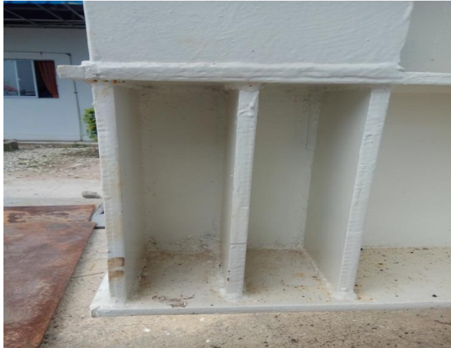
Gambar 2. 102 Tripping Flat bar
