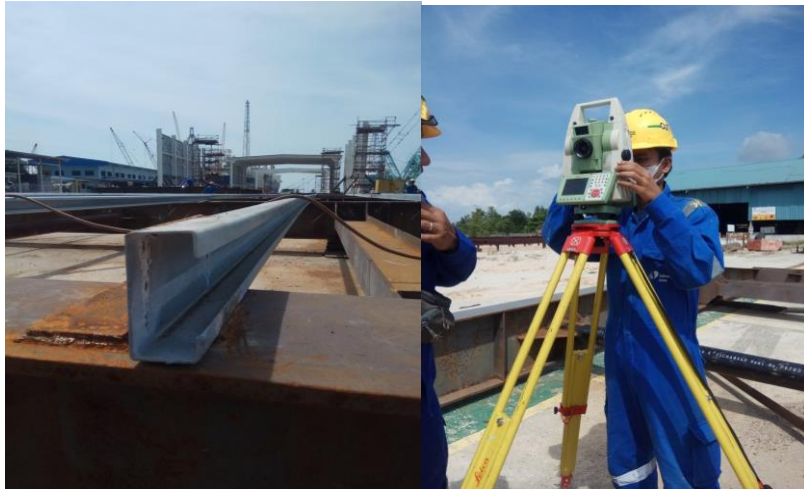
Gambar 2. 95 proses pengukuran dimensi after welding
