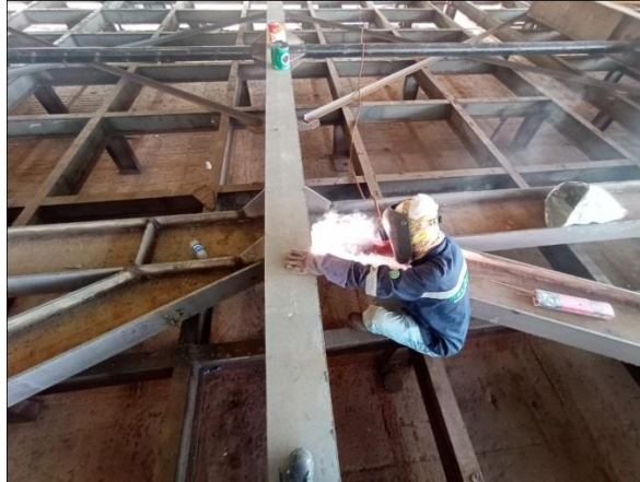
Gambar 2. 108 Proses welding
