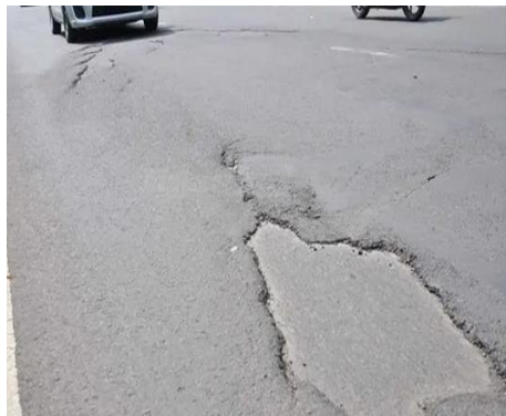
Gambar 2. 20 Stripping (Sumber: Bina Marga, 1990)
