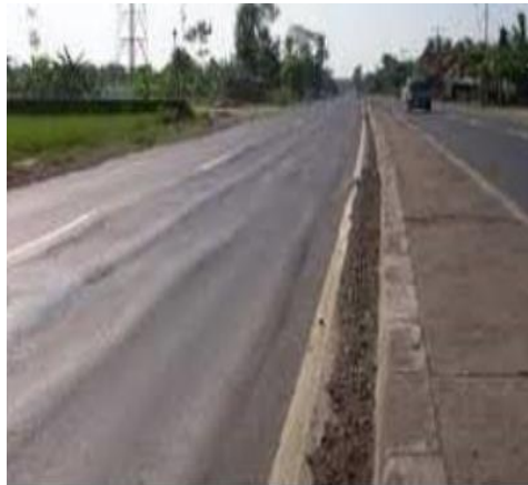
Gambar 2. 11 Alur (Rutting) (Sumber: Bina Marga, 1990)
