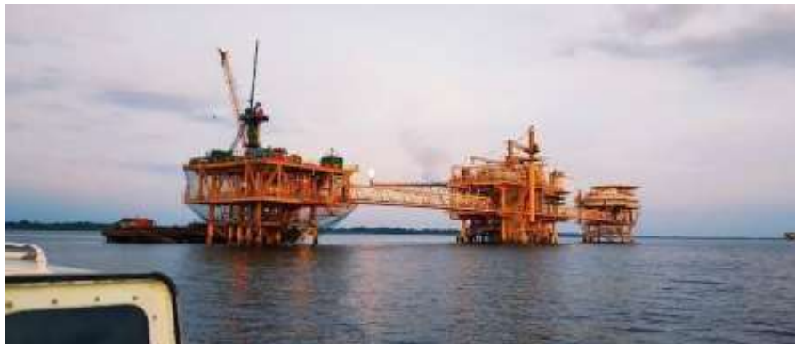
Gambar 2.2 Well Lalang Platform Sumber : PT.Imbang Tata Alam (2023)
