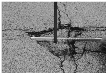
Gambar 2. 7 Lubang ( Pothole )
