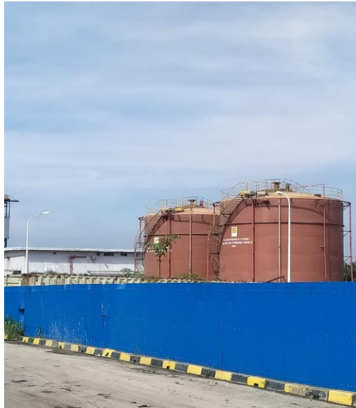
Gambar 2.27. Fuel Oil Tank
