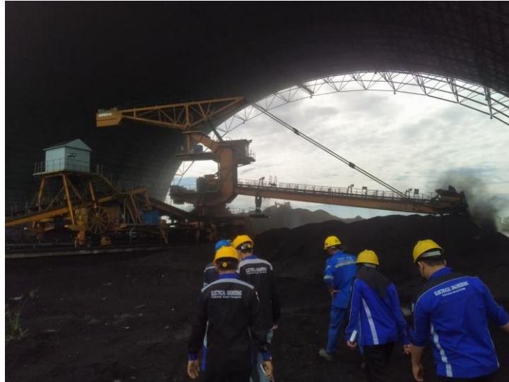
Gambar 2.23. Coal Yard PLTU Tenayan
