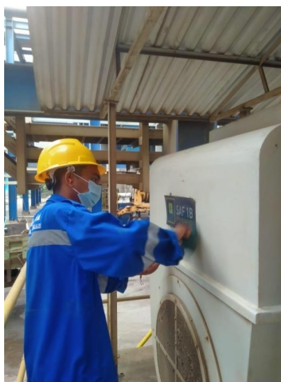
Gambar 2.33. PM Diarea Boiler Motor SAF 1B
