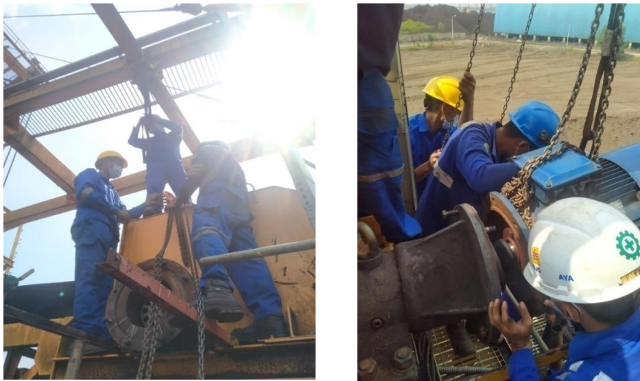
Gambar 2.41. Proses Pemasangan Motor Belt star up 380V Diarea Ship Unloading
