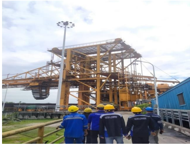
Gambar 2.21. Ship Unloader PLTU Tenayan
