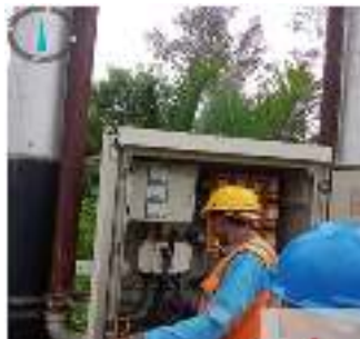
Gambar 2.20 Inspeksi Gardu Distribusi ( Sumber : PT. Adra gemilang, 2023)
