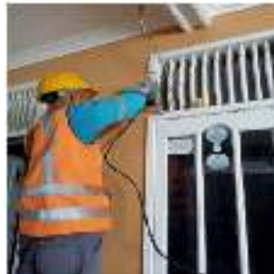
Gambar 2.24 Pergantian KWH Meter ( Sumber : PT. Adra gemilang, 2023)
