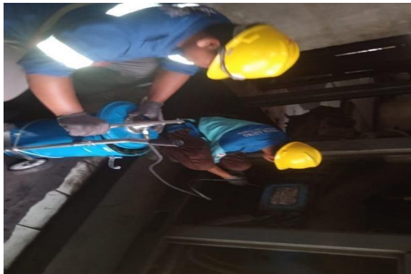
Gambar 2. 45 Greasing Motor Compressor (Sumber: Dokumentasi di PT. Indah Kiat Pulp and Paper)
