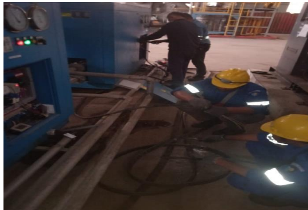
Gambar 2. 37 Tarik Kabel Temporary PG 3 (Sumber: Dokumentasi di PT. Indah Kiat Pulp and Paper)
