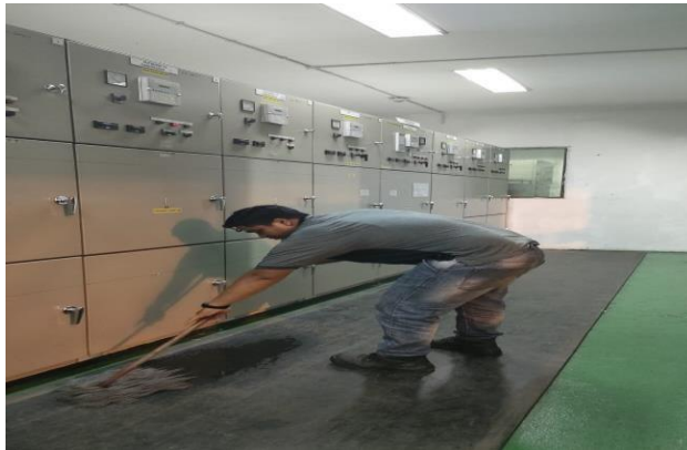
Gambar 2. 20 Celining MCC Room PG 2
