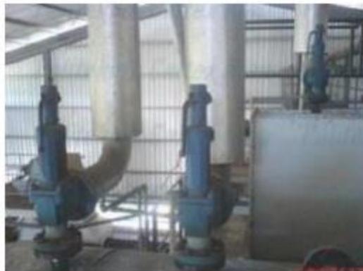
Gambar 3.22 Safety Valve Boiler
