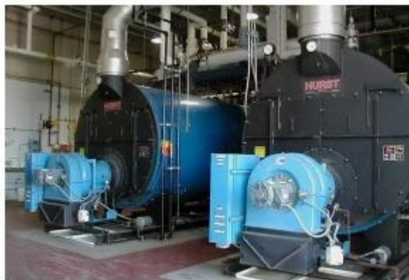
Gambar 3.23 Shoot Blower Boiler
