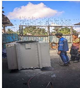
Gambar 2.14 Repaint Body Trafo 1 MVA (Sumber : Dokumentasi 2023)
