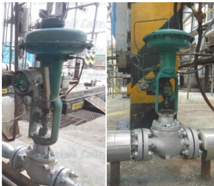
Gambar 3.11 Control Valve ATO dan ATC
