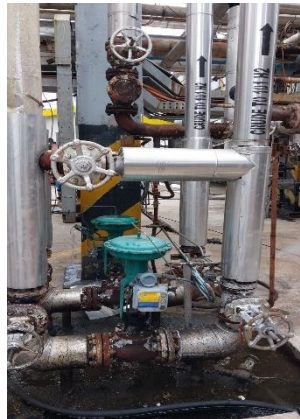
Gambar 3.9 Bukaannya Control Valve Saat Stroke Valve 0%
