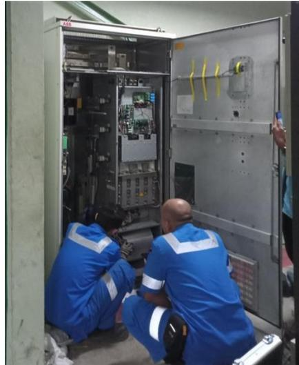
Gambar 2. 26 Penggantian *fan drive* Pulp dryer 1
