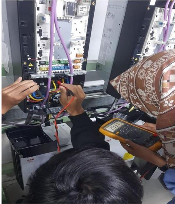
Gambar 2. 10 Gambar Check IGBT
