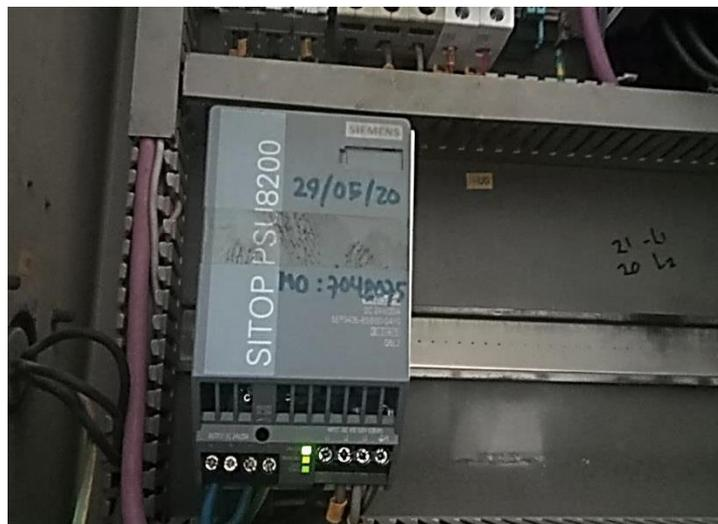
Gambar 3. 5 *Power Supply PLC Siemens*
