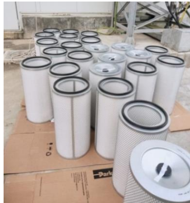
Gambar 3.12 Penggantian filter turbine unit 11
