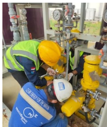
Gambar 3.11 Troubel shooting motor For NaOCL Pump B (Sumber : Dokumentasi pribadi)
