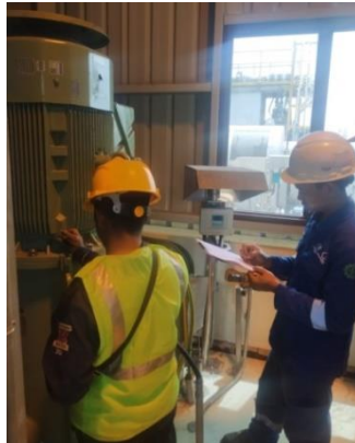
Gambar 3.6 Weekly Inspection River Wwater Intake (RWI)
