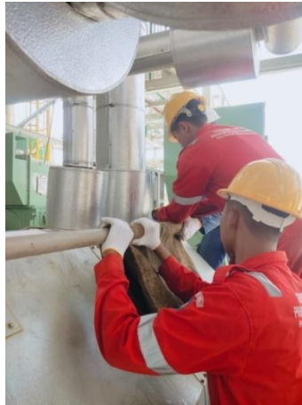
Gambar 3.14 Boiler water feed pump (HRSG unit 11
