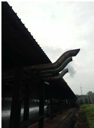
Gambar 3. 14 Saluran Safety Valve
