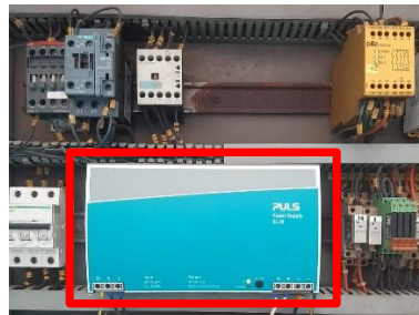
Gambar 3. 14 Power supply pada Folding Machine (Sumber: PT. Riau Andalan Pulp and Paper )
