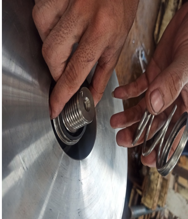
Gambar 4. 21 Pemasangan Mechanical Seal Stationary
