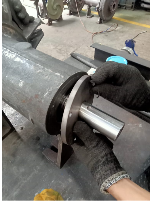
Gambar 4. 19 Pemasangan Bearing Cover
