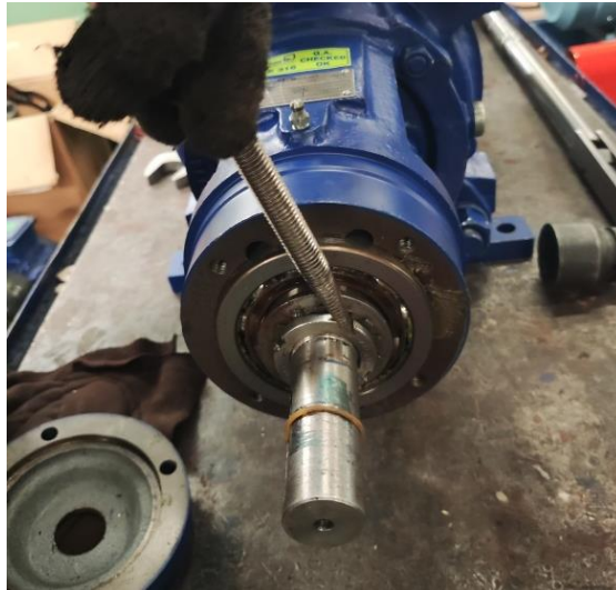
Gambar 4.29 Pemasangan Bearing House Discharge
