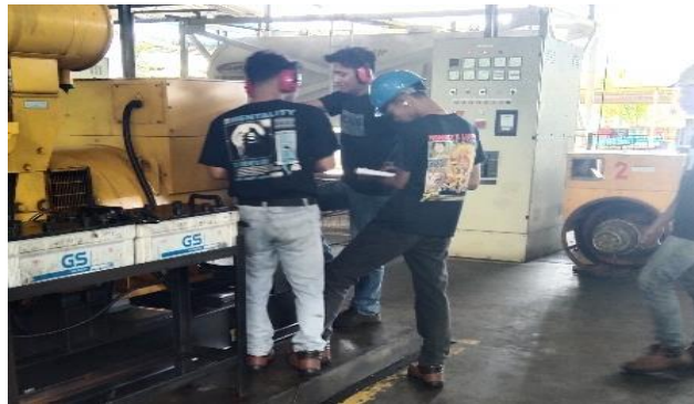
Gambar 2.9 Monitoring kWh (Sumber : PT.Megapower Makmur Tbk,2023)
