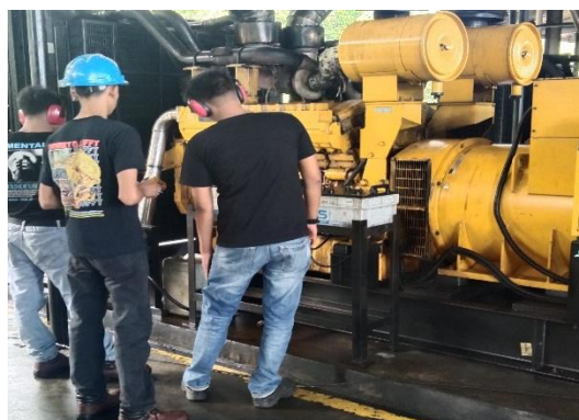
Gambar 2.18 Monitoring kWh (Sumber : PT.Megapower Makmur Tbk,2023)
