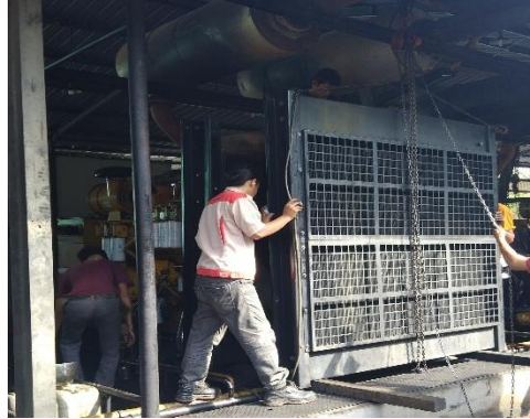
Gambar 2.22 Mengganti radiator unit 3 (Sumber : PT.Megapower Makmur Tbk,2023)
