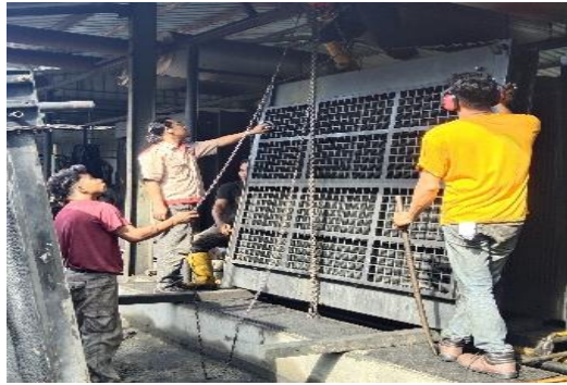
Gambar 2.6 Mengganti radiator (Sumber : PT.Megapower Makmur Tbk,2023)
