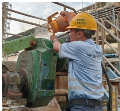
Gambar 4.22 Penambahan Oil Gearbox
