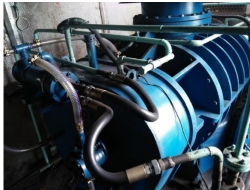
Gambar 4. 1 HIGH PRESSURE FLUIDIZING FAN (HPFF) Sumber: INSTRUKSI KERJA (IK) b PJB-IMS 2.0
