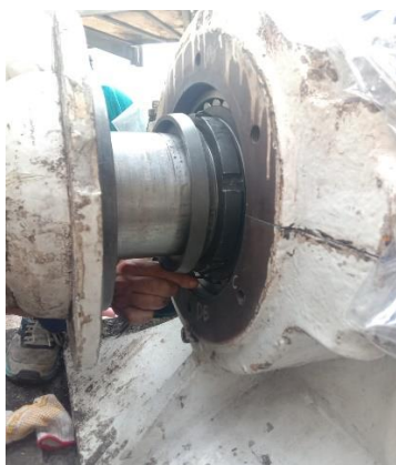
Gambar 4. 40 Pengecekan celah bearing
