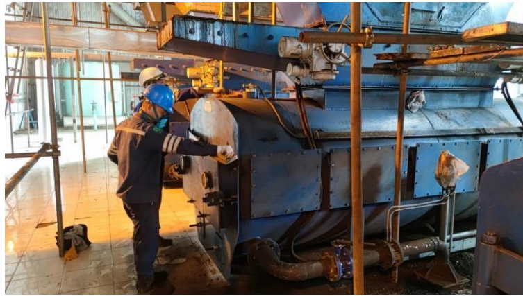
Gambar 3. 1 PM di area coal feeder
