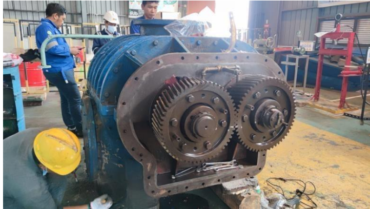
Gambar 3. 4 Perbaikan HPPF (High Pressure Feed Fan)
