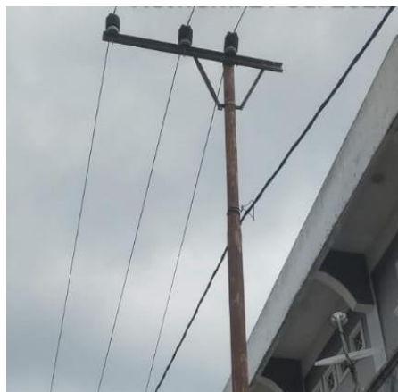
Gambar 4.3.3.a Cross Arm Miring (Sumber: PT. PLN PERSERO ULP DURI, 2023)
