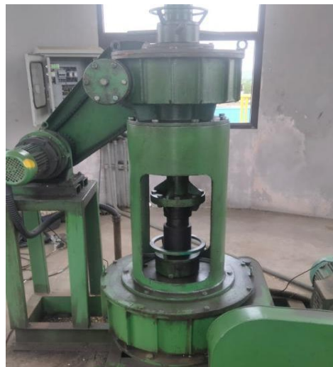
Gambar 3.5 Preventive Maintenance di clarifire (Sumber : Dokumentasi Pribadi)
