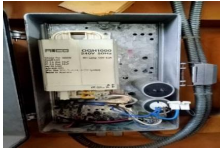
Gambar 2.29 Panel Lighting Crane
