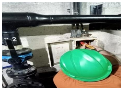
Gambar 2.49 Panel Draniage pump 2.2
