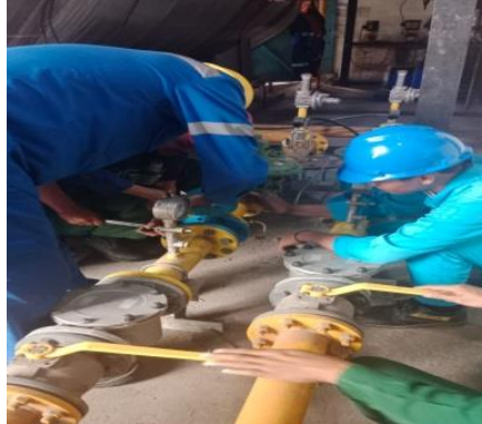
Gambar 2.10 Pengecekan Flowmeter Gas Boiler Advant Sumber: (Dokumentasi, 2023)
