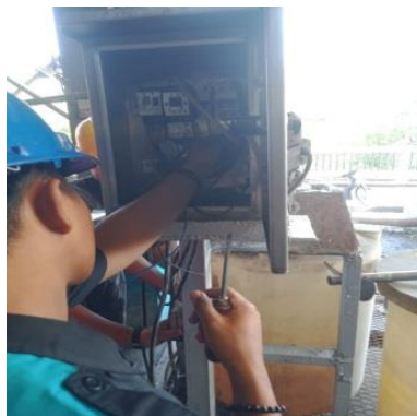
Gambar 2.62 Connect Kabel di Panel Chemical Sumber: (Dokumentasi, 2023)
