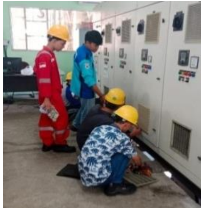
Gambar 2.28 Cleaning Panel di Boiler Sumber: (Dokumentasi, 2023)
