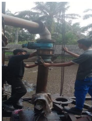
Gambar 2. 49 Penggantian elmots rau water pump
