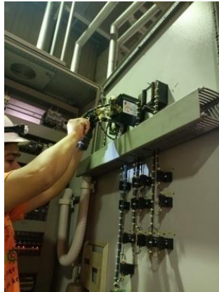
Gambar 2.27 Pengantian Controller Hot Oil Mrek Jumo
