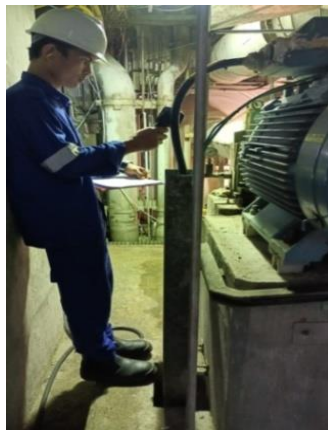
Gambar 2.49 Pengecekan Temperature Motor (Sumber: Dokumentasi PT. Riau Andalan Pulp and Paper Pangkalan Kerinci, 2023)
