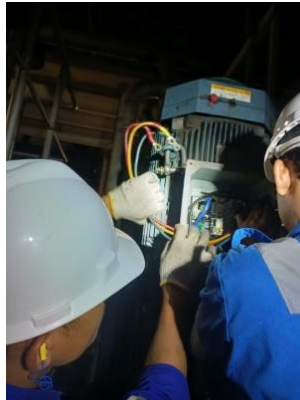
Gambar 2.23 Koneksi Motor Vacuum Pump
