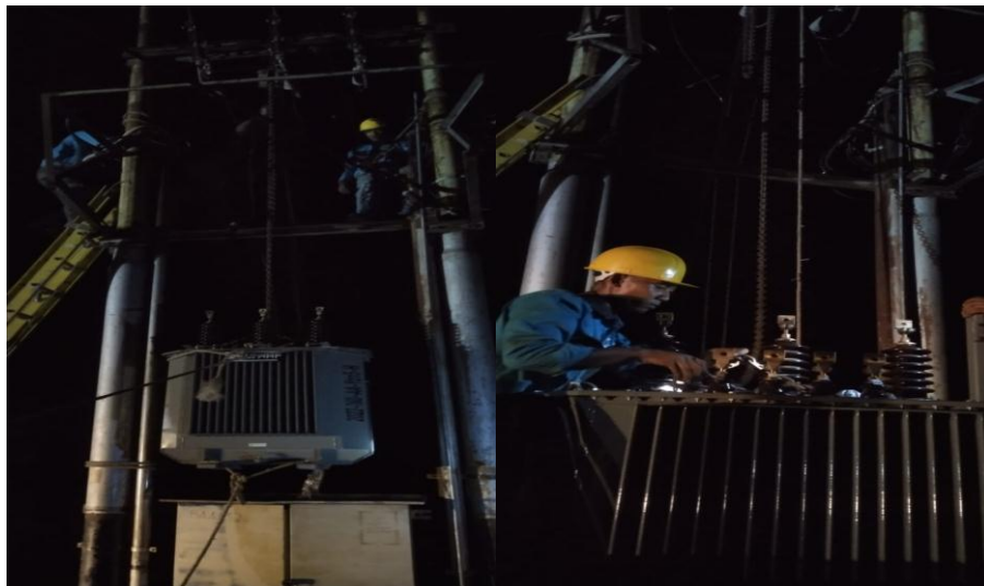
Gambar 3. 13 Penggantian Transformstor
