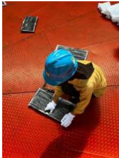
Gambar 2.20 Pergantian filter slip ring
