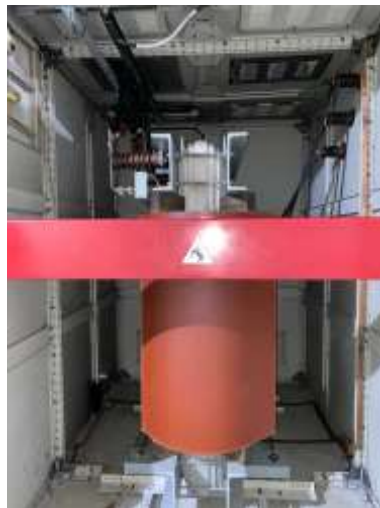
Gambar 4.3 Excitation Transformer
