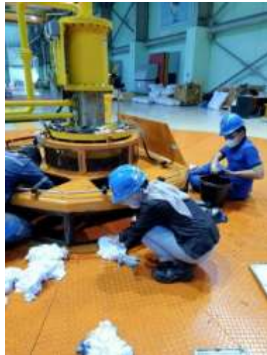
Gambar 2.3 Pergantian Carbon Brush
