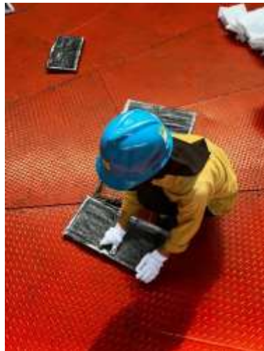
Gambar 4.13 Pergantian filter Slip Ring
