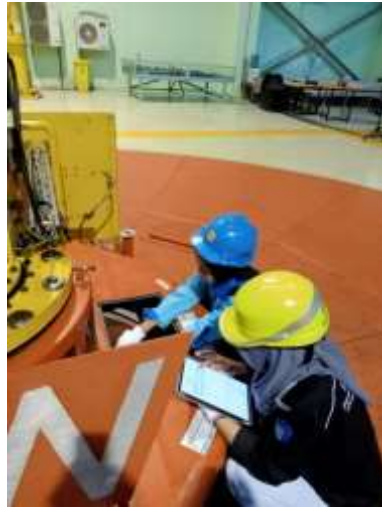
Gambar 2.19 Pengukuran carbon brush
