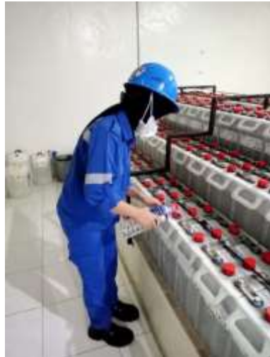
Gambar 2.22 Pengisian accu water
