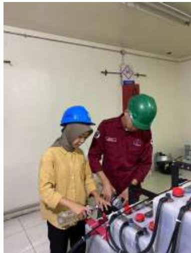
Gambar 2.43 Pengisian accu water
