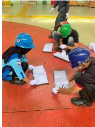
Gambar 2.10 Penggantian Filter Slip Ring
