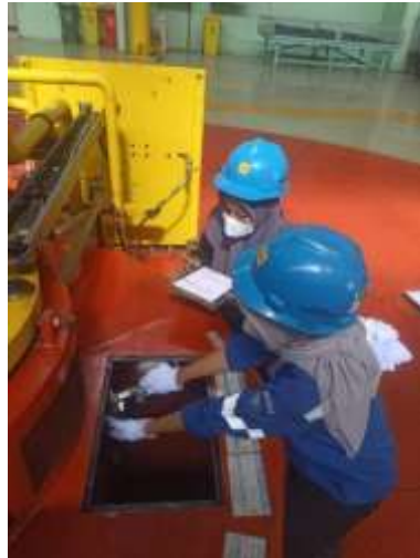
Gambar 2.40 Pengukuran Carbon Brush
