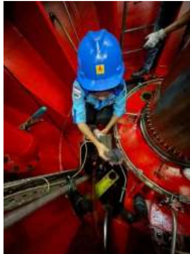
Gambar 2.29 Maintanance Level Switch
