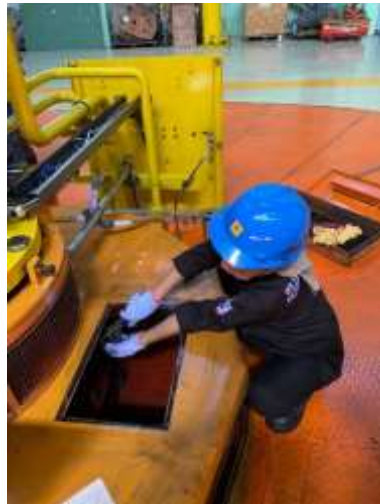
Gambar 4.11 Pengukuran Carbon Brush
