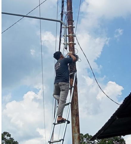
Gambar 3.3 Pengecekan ODP ( Optical Distribution Point )
