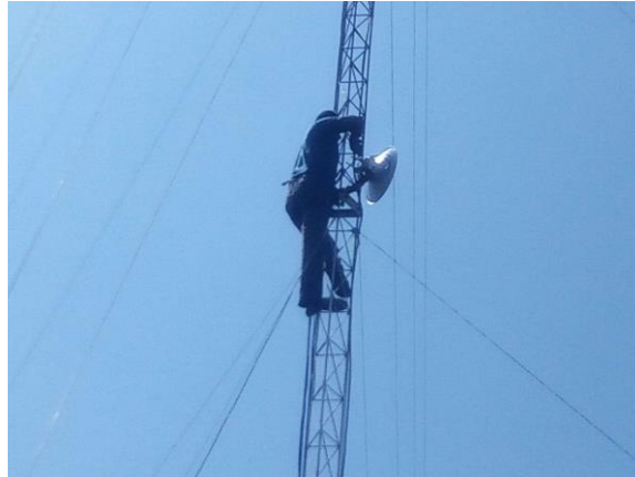
Gambar 3.14 Mempointing Antena LDF
