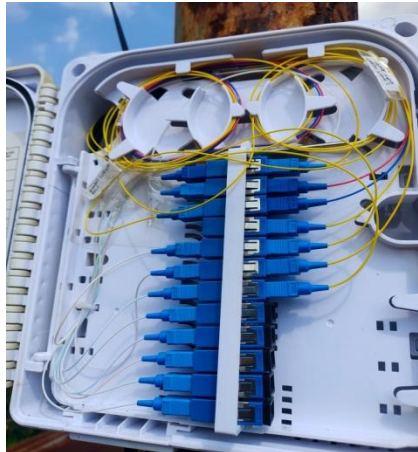
Gambar 4. 3 Optical Distribution Point (ODP)
