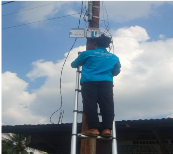
Gambar 3. 3 Pengecekan ODP (Optical Distribution Point)
