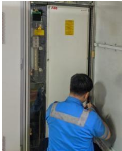
Gambar 2.8 Cleaning Drive fiberline 2 dan 3
