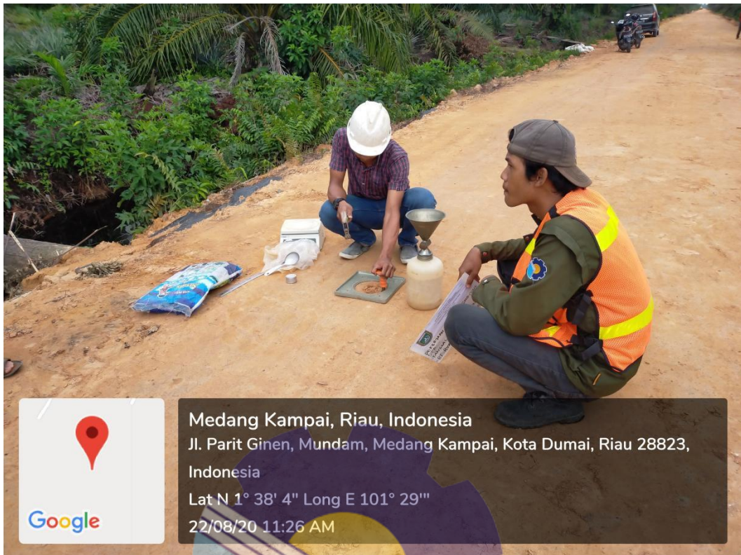
Gambar 4.12 Uji Sand Cone
