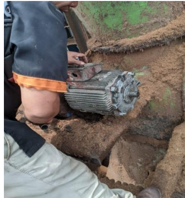
Gambar2. 55 Memasang motor air lock fiber skill
