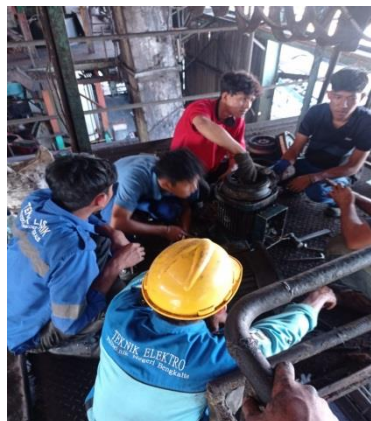
Gambar2. 62 Membongkar motor crane
