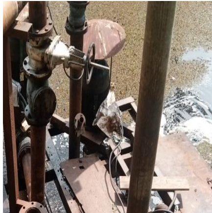
Gambar2. 51 Memasang motor raw water
