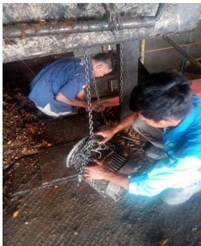
Gambar2. 40 Memasang motor conveyor
