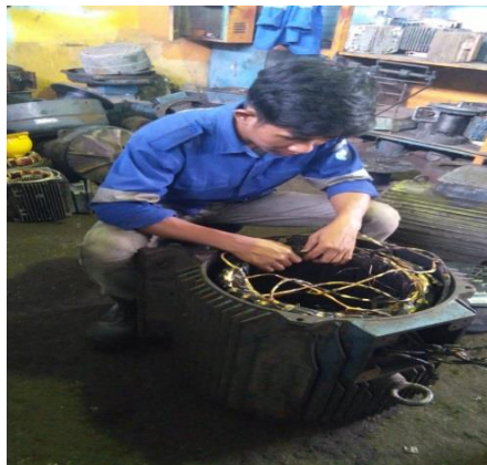
Gambar2. 35 pembongkaran motor denver cover fan
