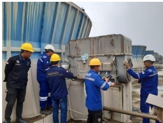
Gambar 2.37 Regreasing cooling tower (Sumber: Dokumentasi 2023)
