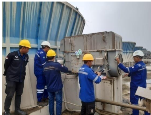
Gambar 2.43 Regreasing cooling tower (Sumber: Dokumentasi 2023)
