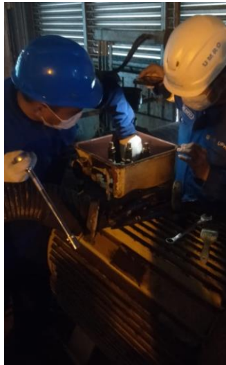
Gambar 2.41 Cleaning & pengecekan motor open cycle cooling water pump 2a (Sumber: Dokumentasi 2023)
