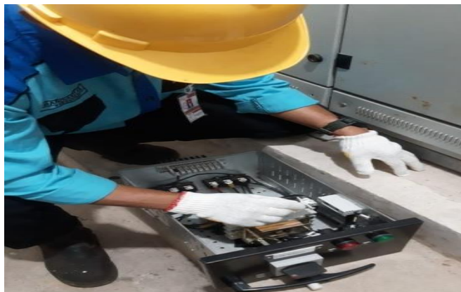
Gambar 2.25 PM PLTU MCC ADMIN BUILDING EL-28D (Sumber: Dokumentasi 2023)
