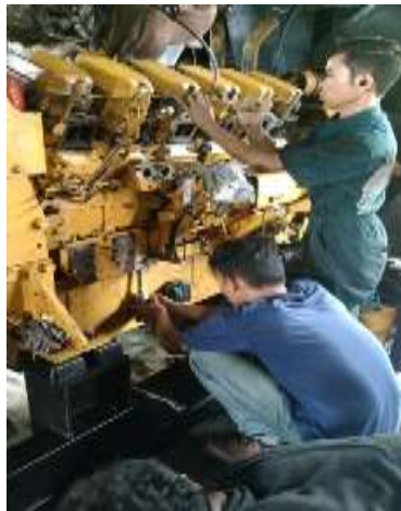
Gambar 2.11 Kegiatan servis mesin unit 5 (Sumber: PT. Megapower Makmur Tbk, 2023)
