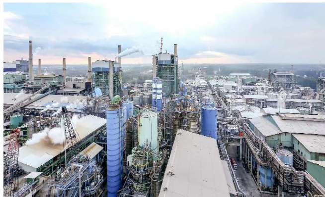
Gambar 1.2 PT. Indah Kiat Pulp and Paper Perawang (Sumber: https://indahkiat.co.id/in/inдах-kiat-perawang )
