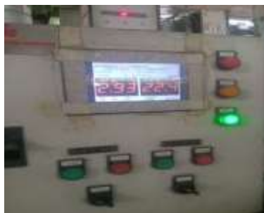
Gambar 2. 21 Monitoring Steam inlet dan Steam Outlet di Kamar mesin Sumber : Dokumentasi 2023
