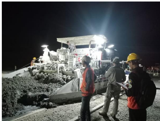
Gambar 3. 47 Penghamparan Beton Rigid Pavement
