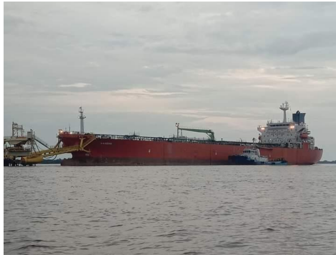
Gambar 1. 4 Terminal unit oil storage tangker (Gandini)
