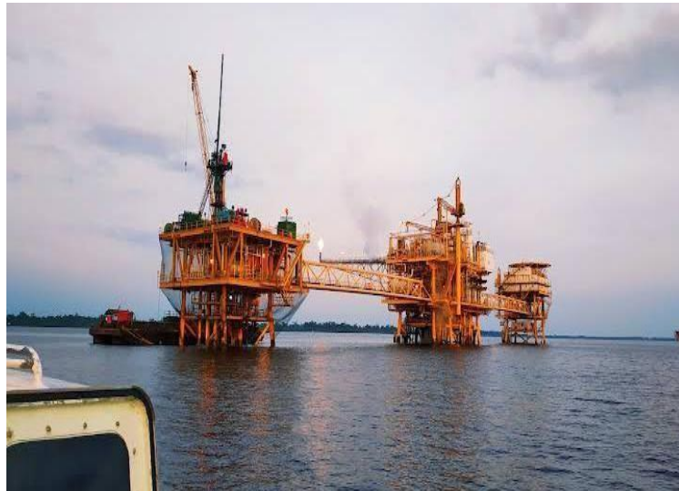
Gambar 1. 3 Well Lalang Platform
