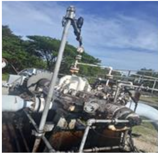
Gambar 4. 2 pompa sentrifugal (COTP)
