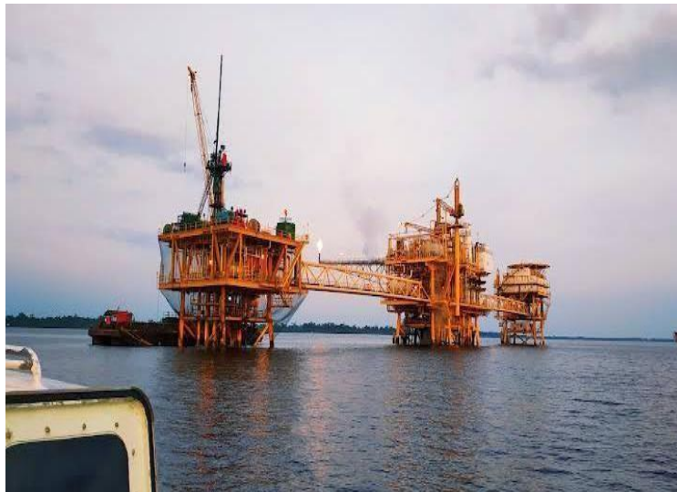
Gambar 2. 3 Well Lalang Platform (Sumber : PT.Imbang Tata Alam 2022)
