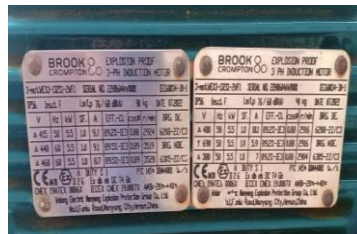
Gambar 3. 3 Nam plate motor 3 phasa (Sumber : PT. Sari Dumai Oleo)
