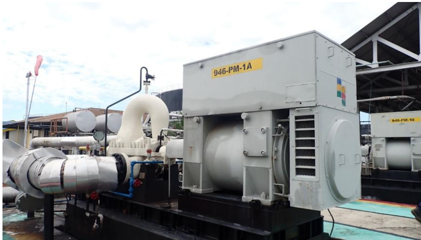
Gambar 4.1 Pompa Feed
