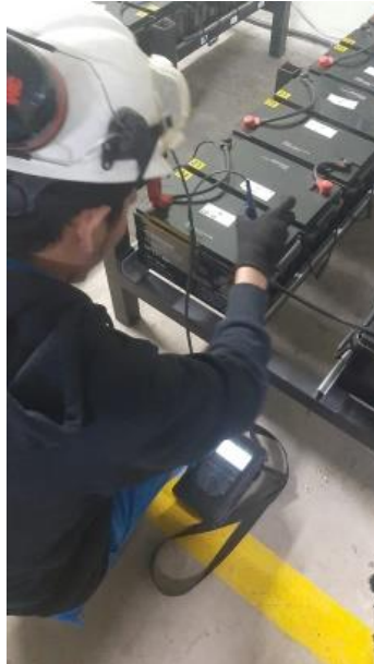
Gambar 2.13 Pengecekan Battery
