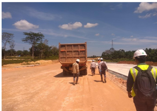
Gambar 3. 18 Pengujian Proof Folling (Capping Layer)
