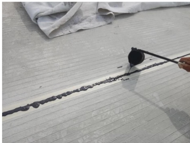
Gambar 3. 66 Pekerjaan Joint Sealent
