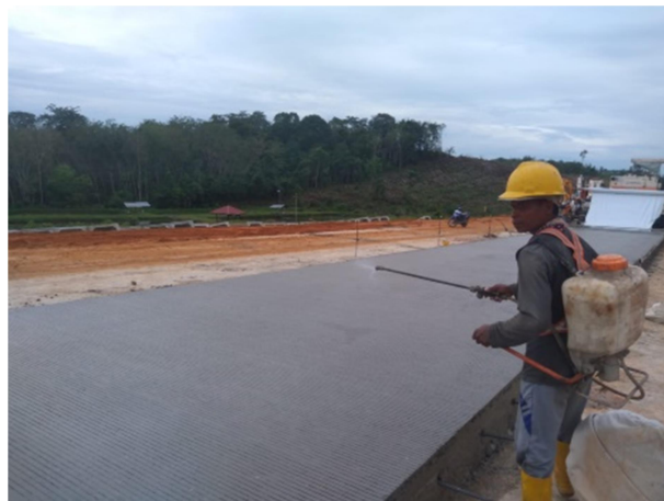
Gambar 3. 44 Pekerjaan Curing Compound rigid
