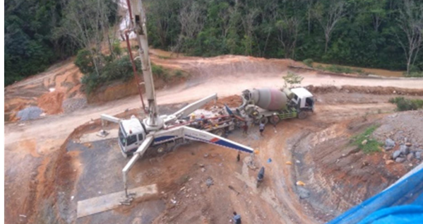
Gambar 3. 12 Persiapan Alat Berat Concrete Pump
