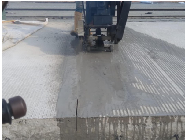
Gambar 3. 65 Proses Cutting
