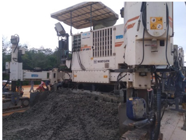
Gambar 3. 57 Proses Kerja Auger
