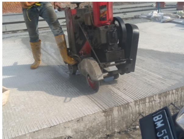
Gambar 3. 46 Pekerjaan Concrete Cutter
