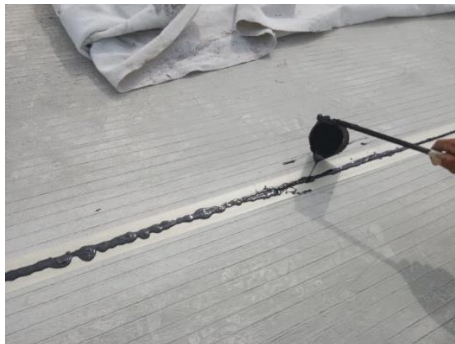
Gambar 4. 21 Pekerjaan joint sealent
