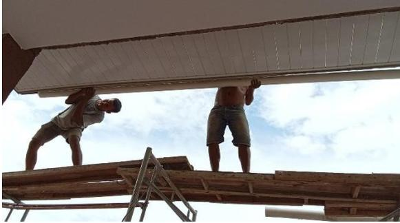
A photograph showing two construction workers on a wooden roof structure. They are working together to install a long, white gutter along the edge of the roof. The sky is visible in the background.               | Proses Pemasangan talang air atap     |
