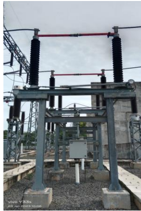
Gambar 3. 4 Disconnecting Switch with Earthing (DS/E) (Sumber : Dokumentasi, 2023)
