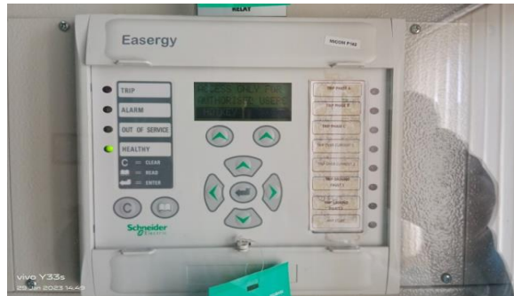
Gambar 3. 10 Over Current relay (Sumber : Dokumentasi, 2023)
